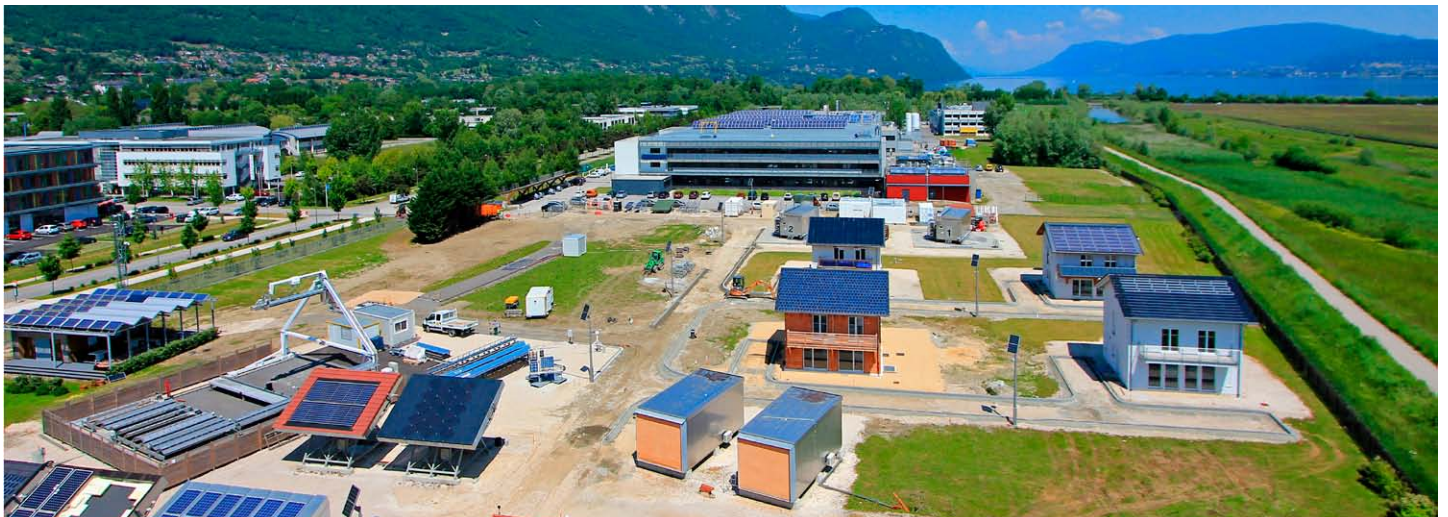
Figure3: INCAS experimental platform of CEA INES, at the middle two PASSYS test cells, at the back INCAS experimental houses
